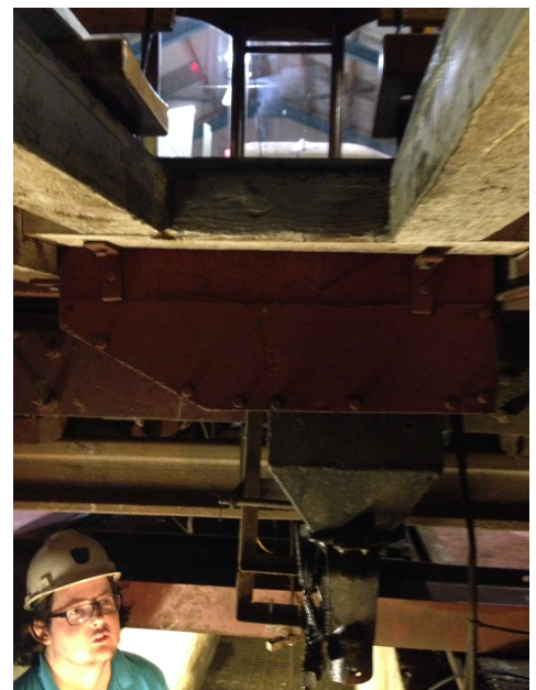
Looking up through 1017s floor. The sandbox can be seen just below the floor
